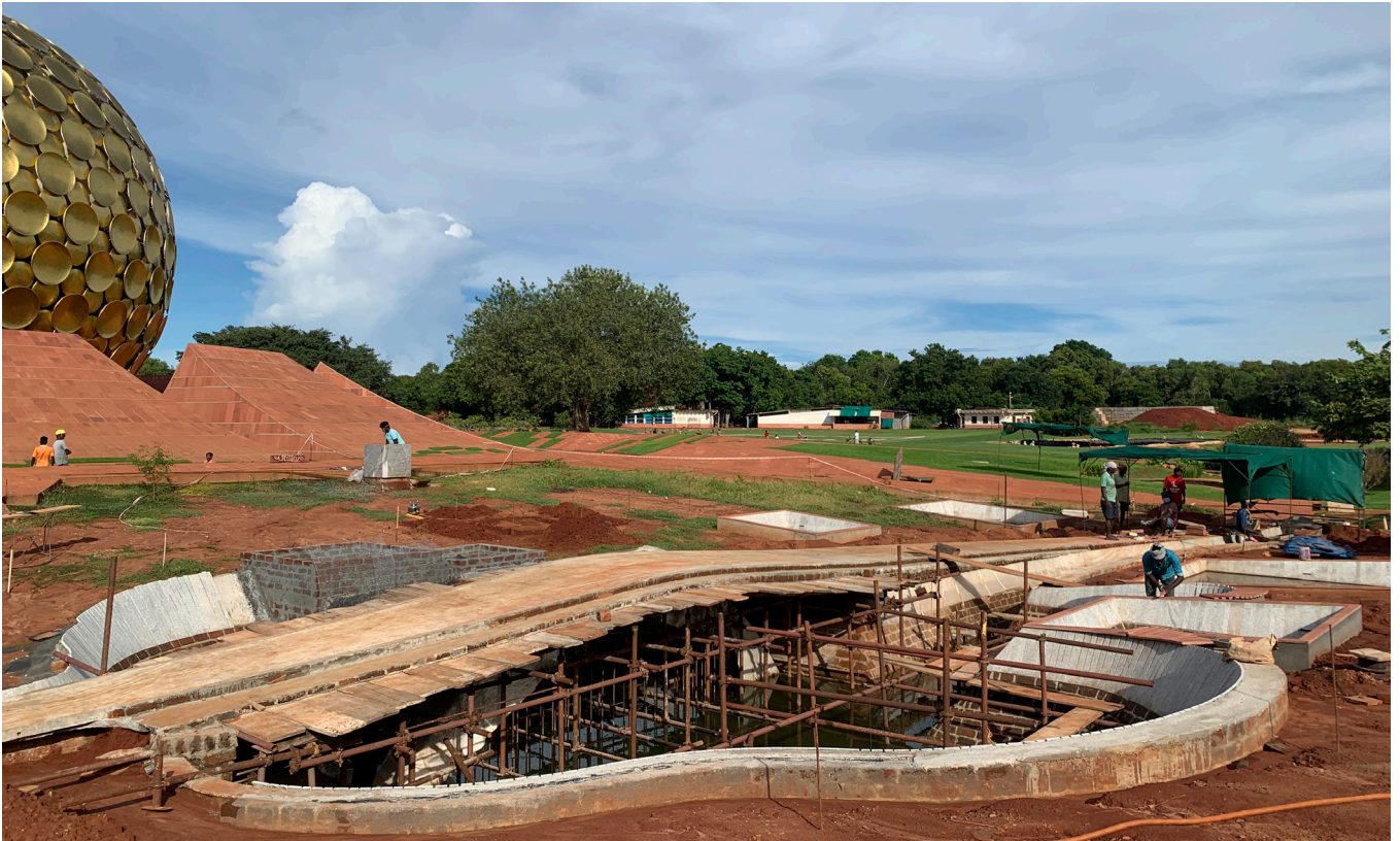
The Garden of Utility under construction
