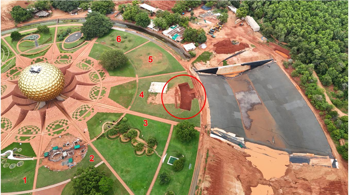
Drone view showing the location of the excavated underground room in the Garden of Youth (4), marked with a red circle. The Garden of Harmony (5) will be built in the plot to the North of the Garden of Youth. Construction activity in the Garden of Utility (2) is seen at the lower left, between the completed Gardens of Wealth (1) and Progress (3). Work on the Garden of Perfection (6) will begin soon.
